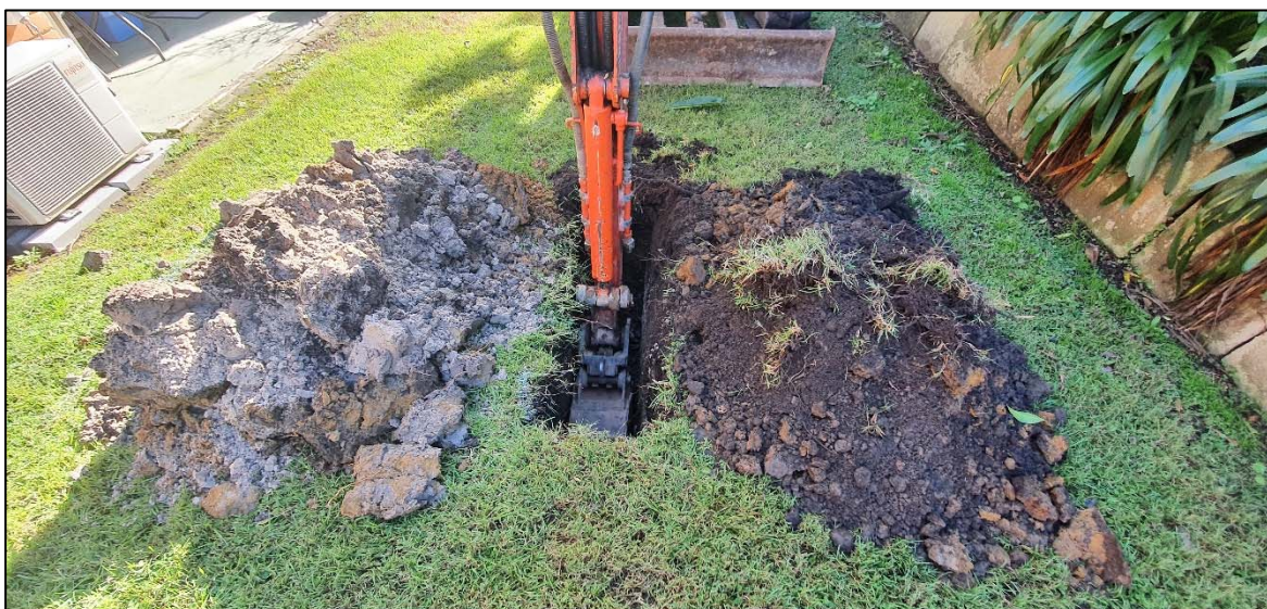
Image 8 View of 3.5t excavator at test pit TP15
